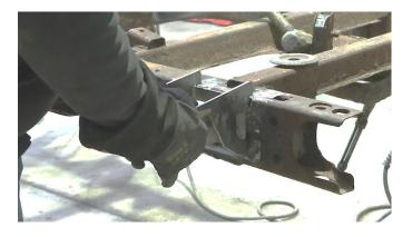
Then, tac weld it into the frame before welding it on fully. Weld 100% around all edges.
