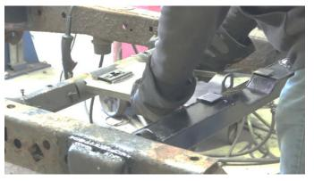
Following proper welding procedures, tac weld your spare tire plate onto the frame before welding it on fully.
